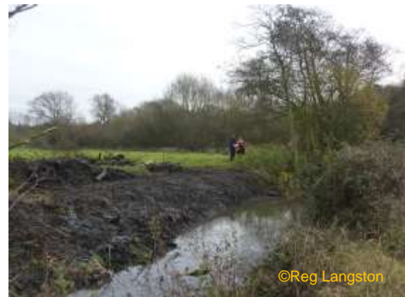
Ditch reprofiling in progress Scarfe Meadows
